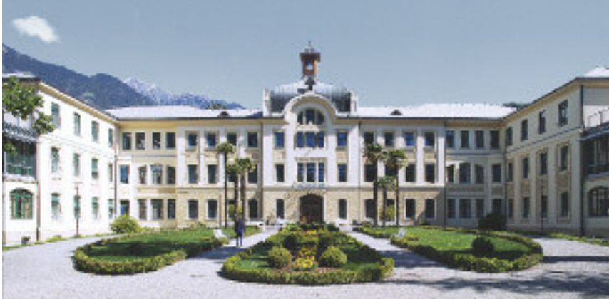
Franz-Tappeiner Krankenhaus Refurbishment, Meran, IT
